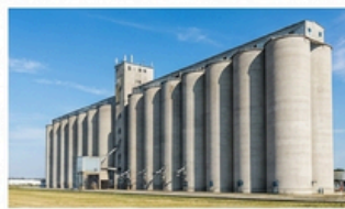
Grain and Cement Storage Silos
